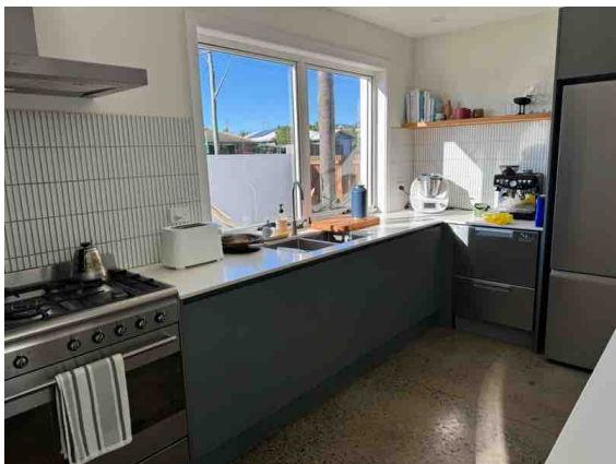
Example of kitchen cupboards and appliances limiting full visual inspection
