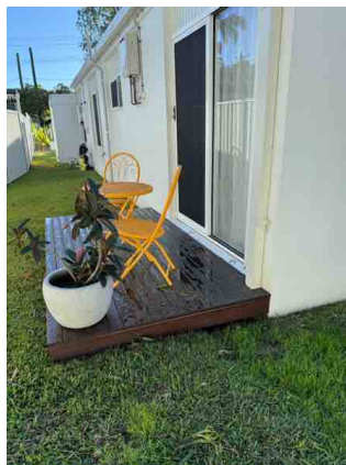
Timber decks conceal base of exterior walls.
